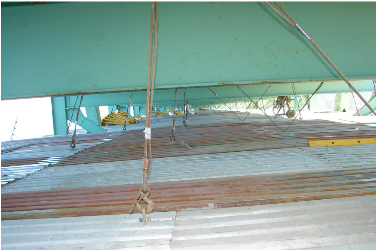
Platform & Tie Ups
