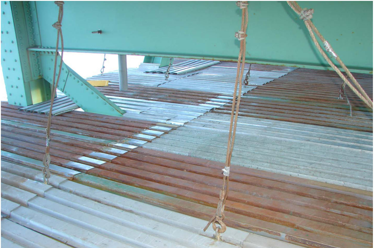
Platform & Tie Ups
