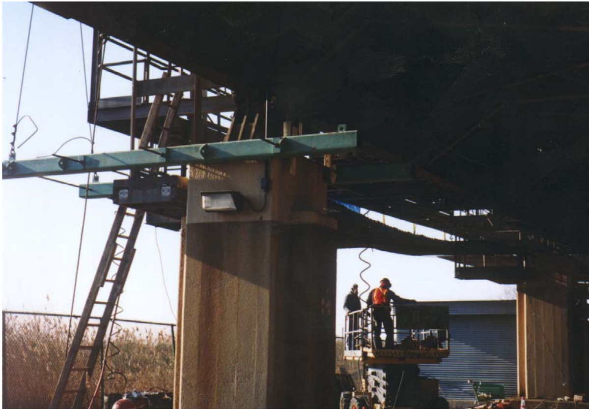
Horizontal Support Tube Column Cap Clamping Assembly
