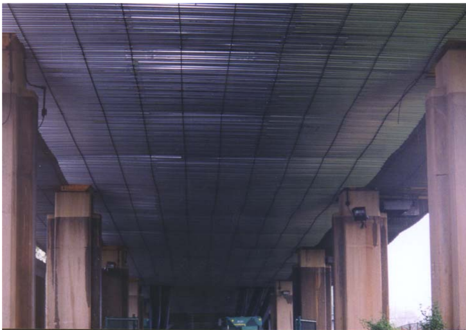
Cable Supported Platform
