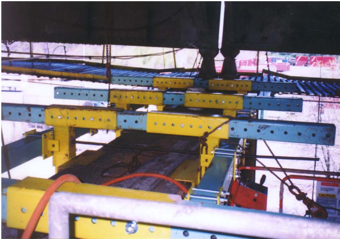
Horizontal Support Tube Pier Clamping Assembly
