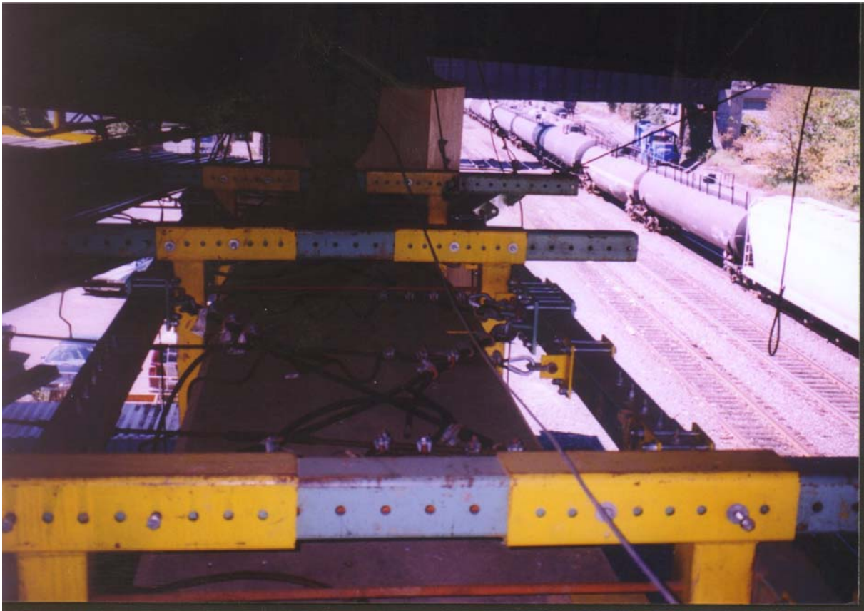
Horizontal Support Tube Pier Clamping Assembly
