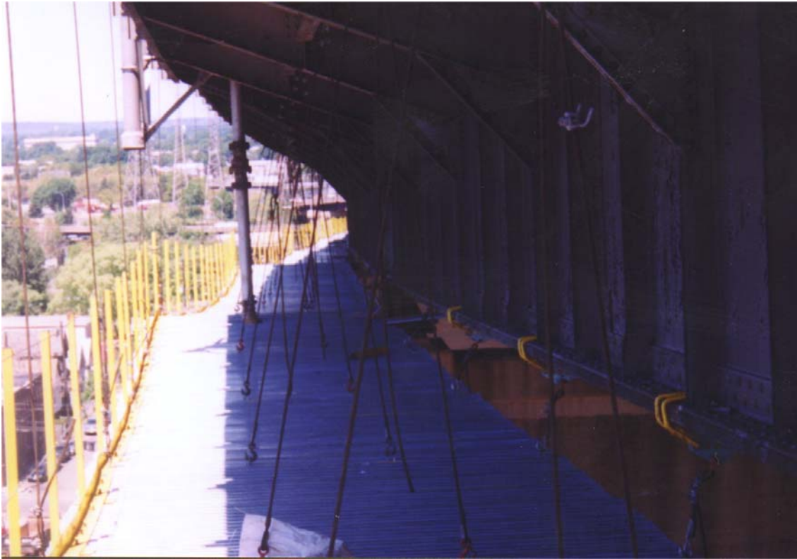
Cable Supported Platform
