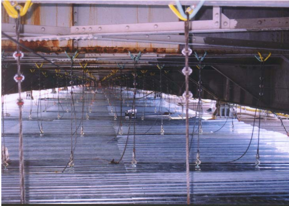
Cable Supported Platform
