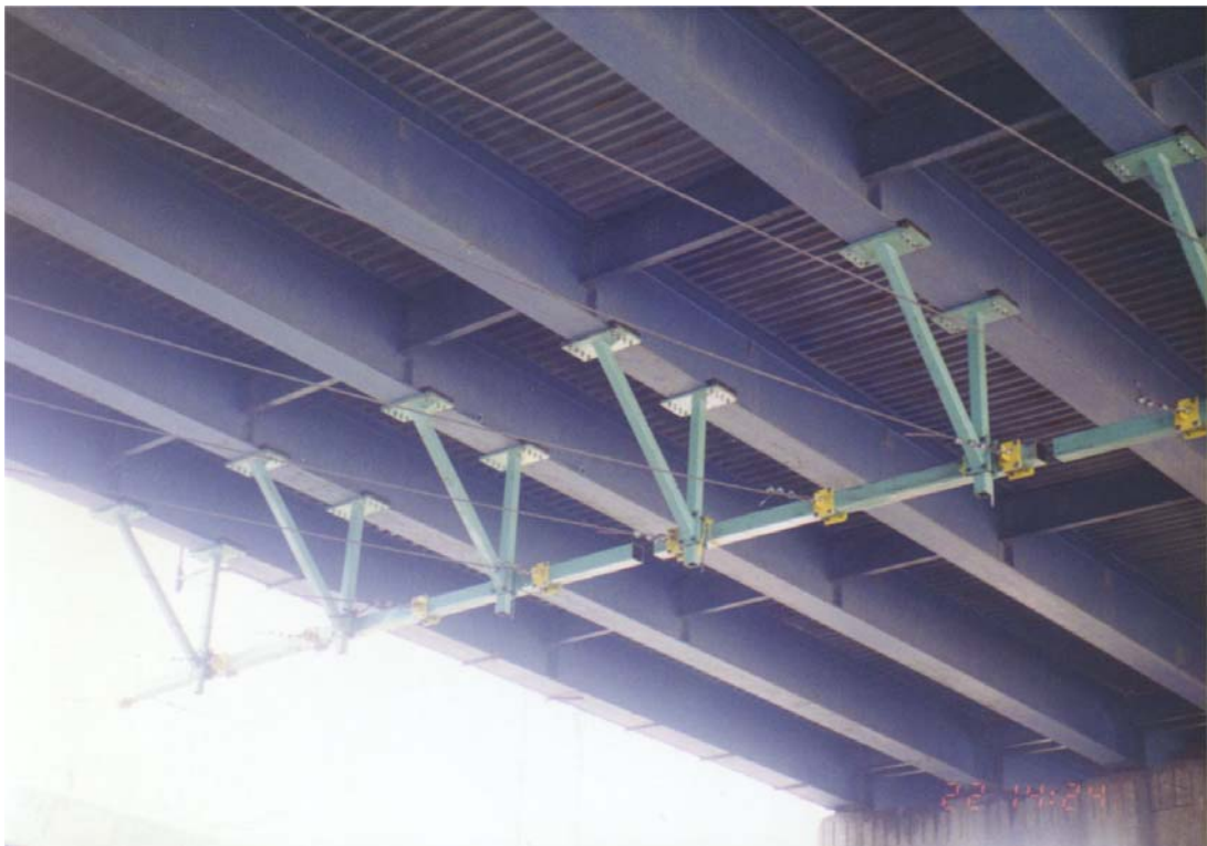
Post Bracket/Horizontal Support Tube End Connection Assembly
