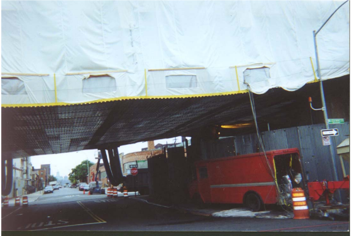
Cable Supported Platform, Perimeter Protection & Containment
