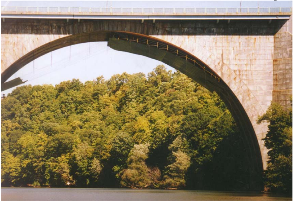
Partially installed Cable/Metal Deck Platform Conforming to the Concrete Arch
