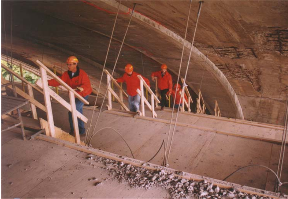
Metal Frame/Plywood Horizontal Work Surface w/Debris Chute in the Center
