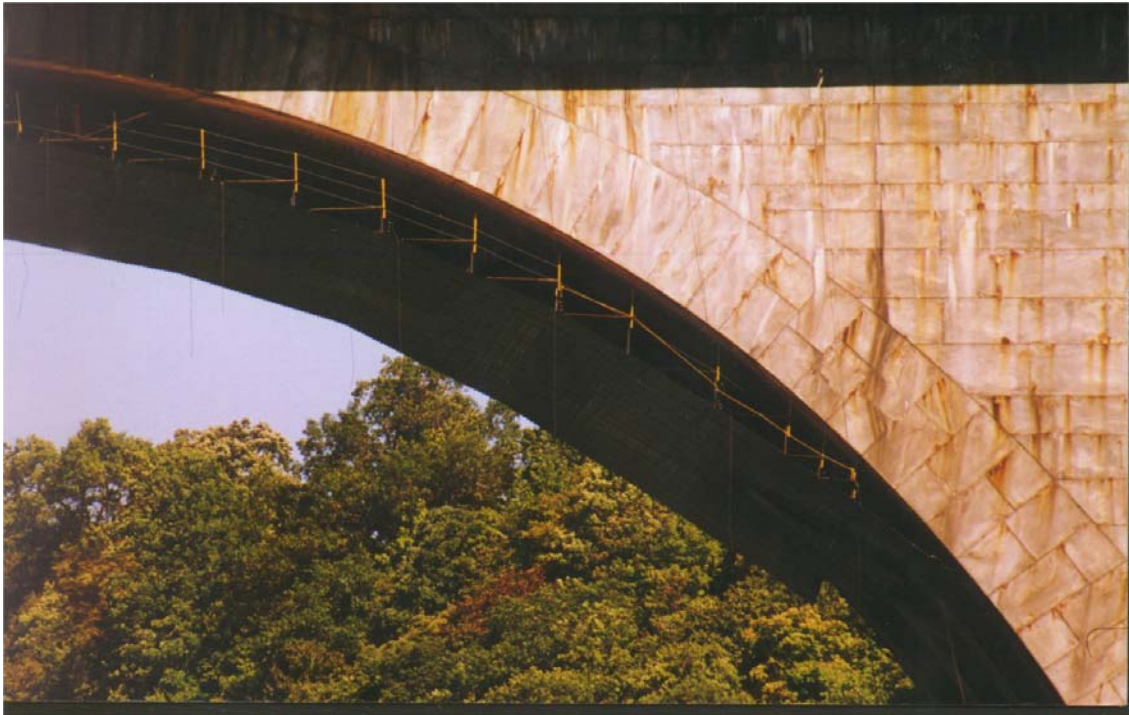
Partially installed Cable/Metal Deck Platform Conforming to the Concrete Arch
