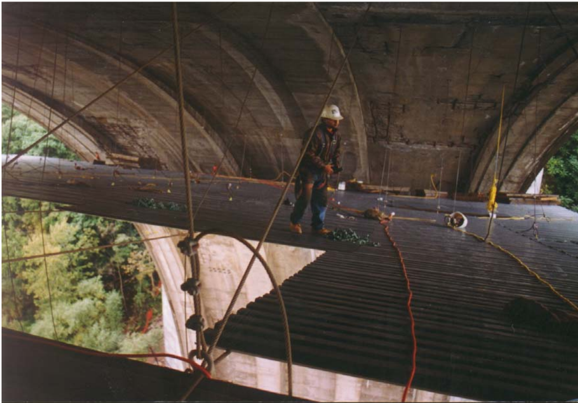
Partially installed Cable/Metal Deck Platform Conforming to the Concrete Arch
