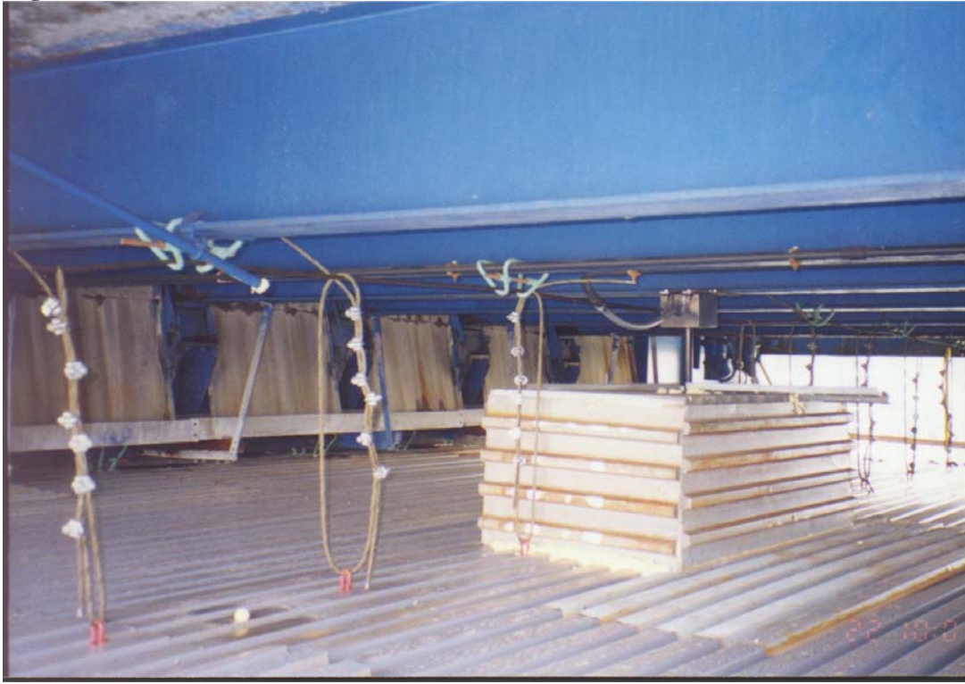
Cable Supported Platform, Tie Ups & Protective Light Box Covers
