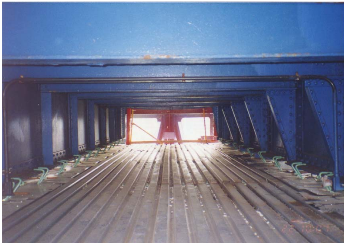
Beam Flange Clamp Hanger Main Cable Support System w/Metal Deck Floor
